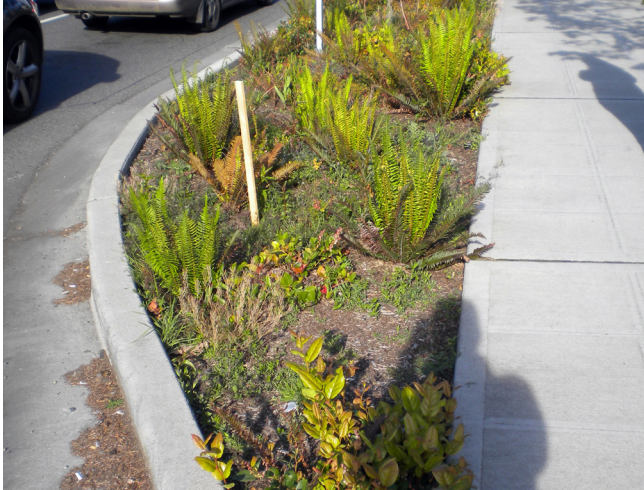
Bioswales planted with native species provide an effective alternative to more expensive concrete drainage infrastructure.
