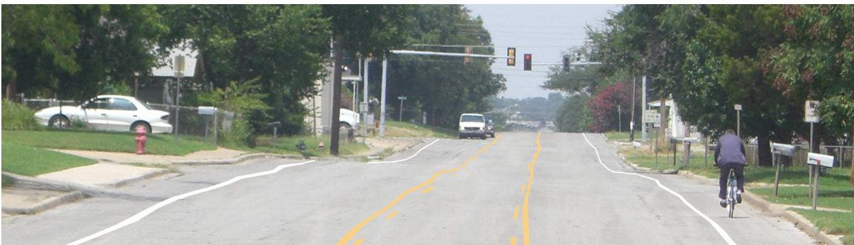
Many four-lane roads within Shreveport have excess capacity and could inexpensively provide safe turn-in and bicycle lanes through restriping—with no increase in congestion.
