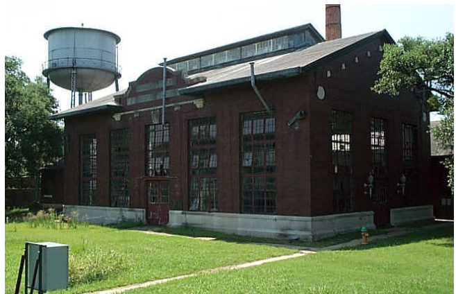
McNeill Street Pumping Station (Shreveport Waterworks Museum) is a National Historic Landmark
