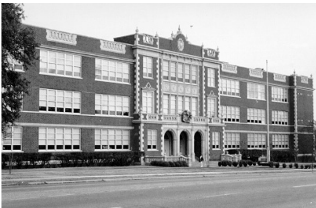
C.E. Byrd High School: An example of the Tudor Revival style of architecture from the early twentieth century.
