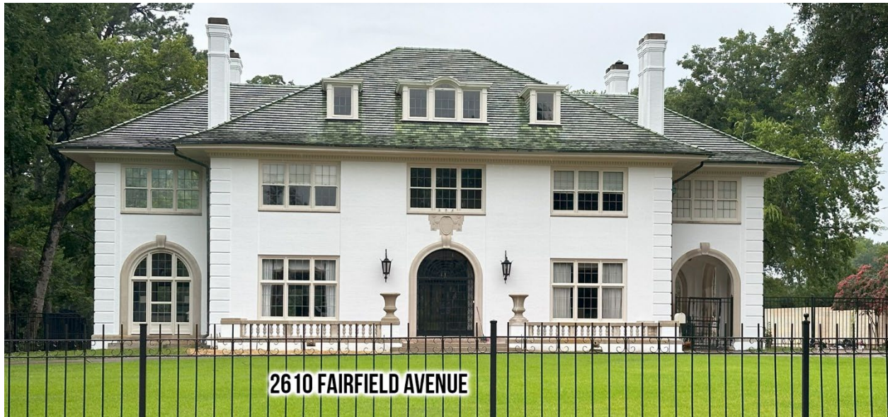
Exhibit A. Front Facade View
