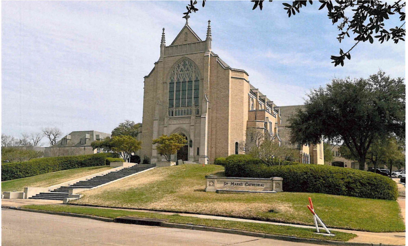
Figure 2. St. Mark's School Entry. Courtyard is in the background, behind the oak tree.
