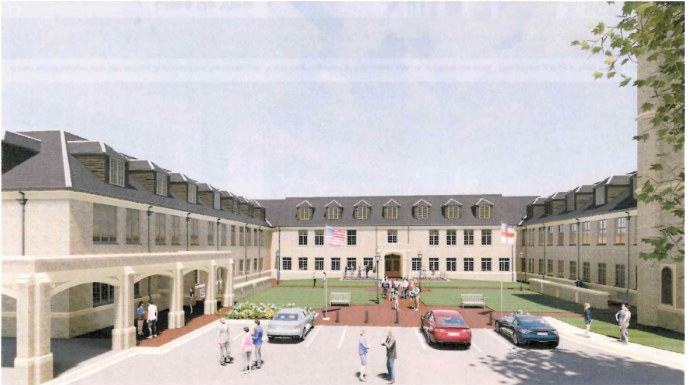
A new columbarium with 384 niches is planned for the courtyard. It will be composed of 8 identical panels of 48 niches each. The panels will be 9' long x 4'-3" tall x 2' wide.
