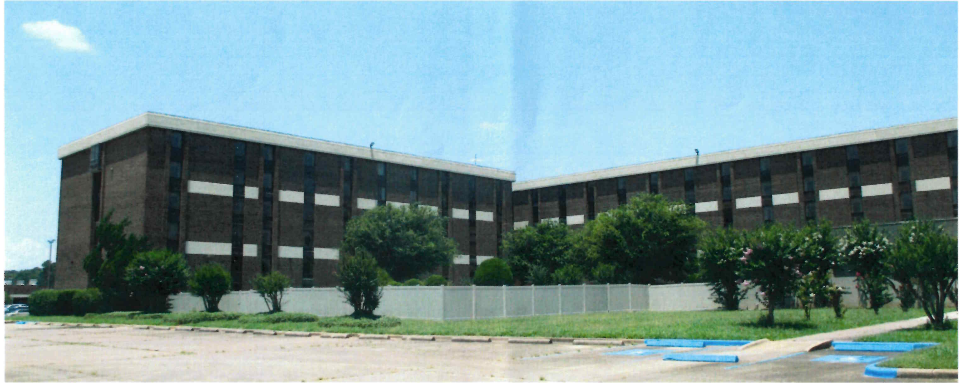
2 EXISTING SOUTHEAST VIEW A0.1B 3" = 1'-0"
