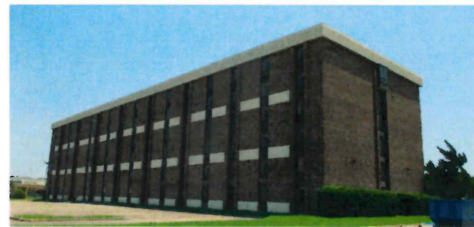
3 EXISTING SOUTHWEST VIEW
